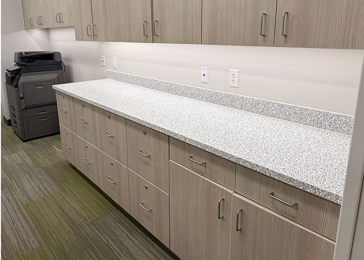
AAPG Plastic-Laminate-Clad Casework — woodgrain HPL-clad wall and base cabinets with a solid-surface countertop in a commercial work room. Project installation shown for reference; laminate color, configuration, and hardware are as specified for that project rather than as documented on this sheet.
